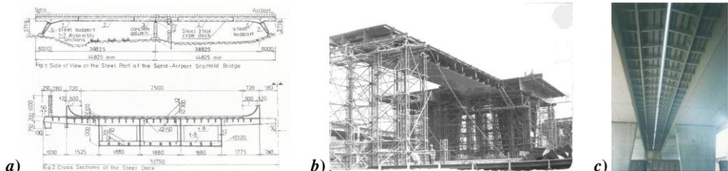
Figure 6a,b,c. “Brussels“ Blvd. steel bridge: Longitudinal and cross-section-a), While erecting the bridge-b), View of the orthotropic bridge-c)
