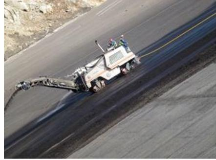
**Fig. 2. Vertical milling of the existing ACF**
