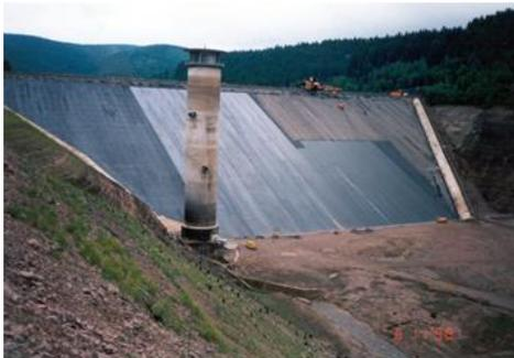
**Fig. 5. Rehabilitation of an asphalt concrete faced dam, vertical placing**
