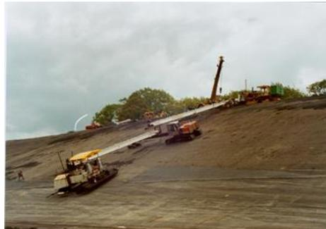
**Fig. 6. Horizontal placing of the new asphalt concrete sealing**
