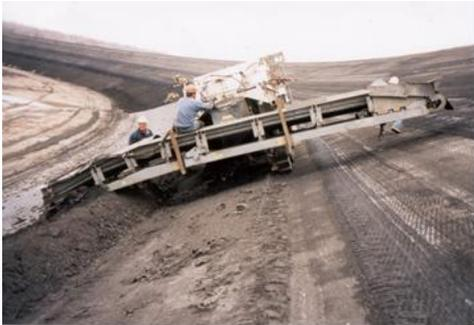
**Fig. 3. Horizontal milling of the existing ACF**
