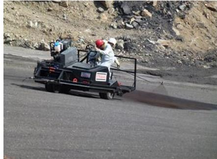
**Fig. 4. Spraying of emulsion on top of the milled surface**
