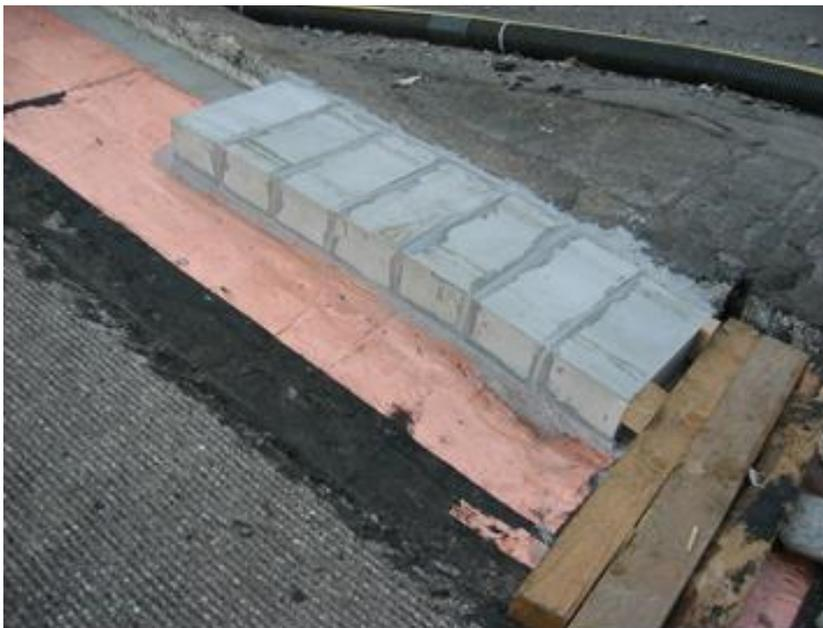
**Fig. 7. Connection between ACF and plinth with copper water stop and bricks**
