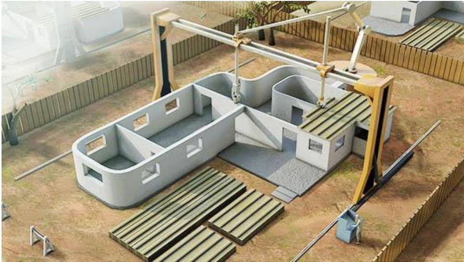
**Figure 3. Contour crafting building printer [3DPrint.com]**
