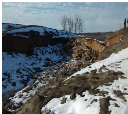
Figure 6. The overflow of the Lesura dam
