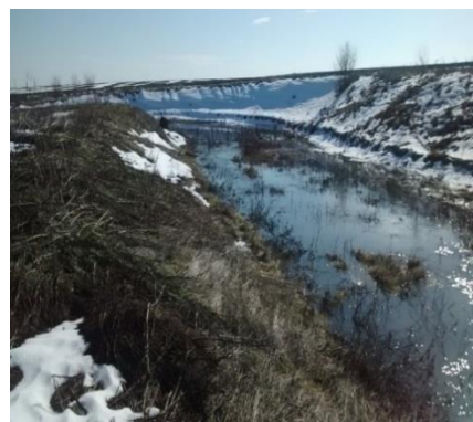
Figure 4. Wire net on the overflow of the Ezerska padina dam
