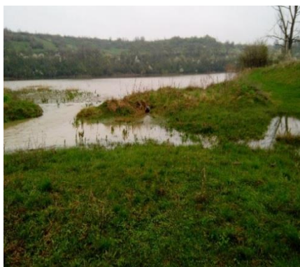
Figure 3. Buried overflow of the Zharkovets dam
