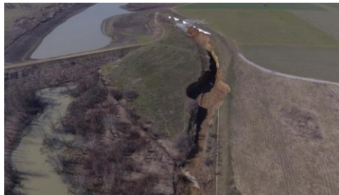
Figure 5. Damage of an eroded chute after spillway
