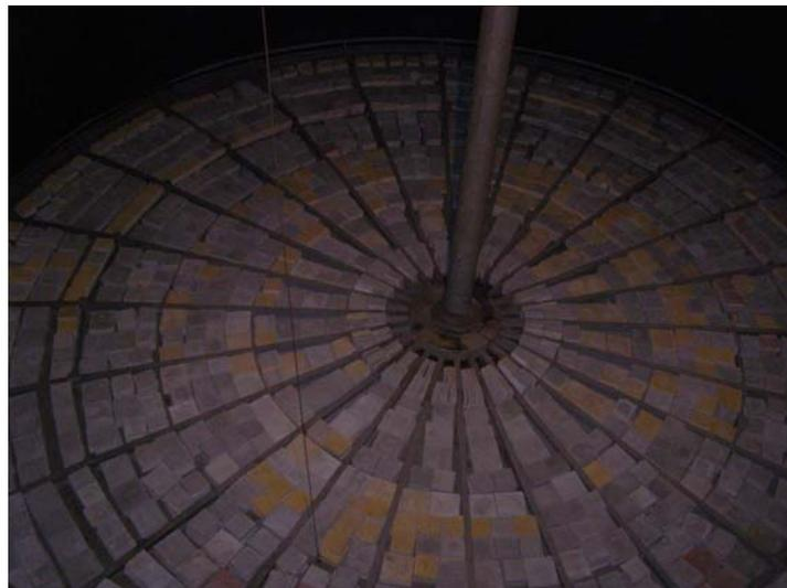
fig. 2 Moving ceiling and central telescopic column
