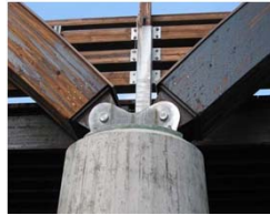
This is the connection at the end of two arcs to the support.
