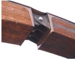
This is the connection in the middle of the bridges arc.
