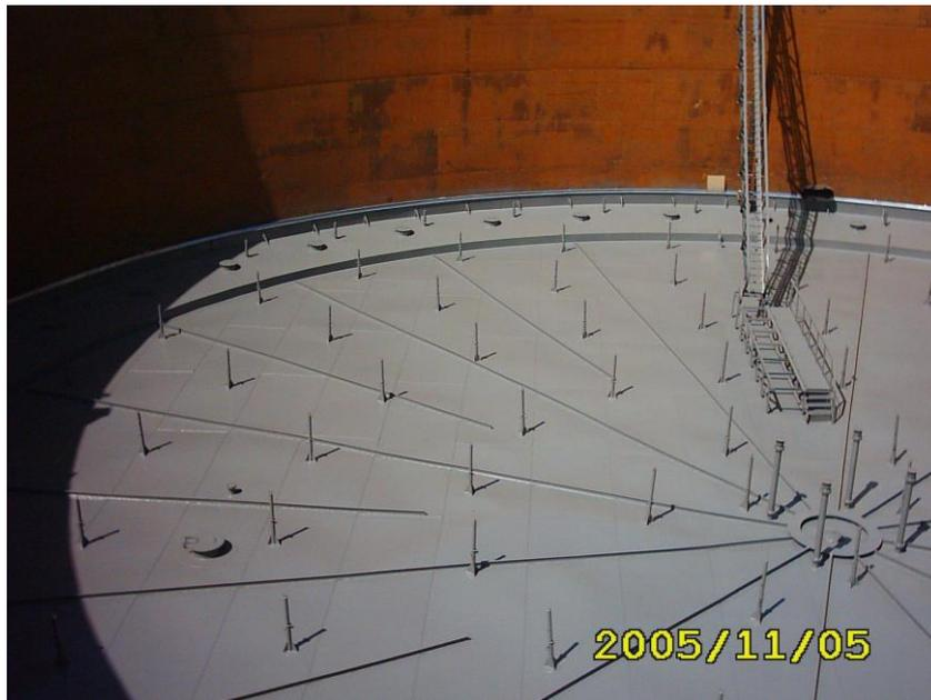
fig. 6 Stiffening of membrane with radial girders, Sudan
