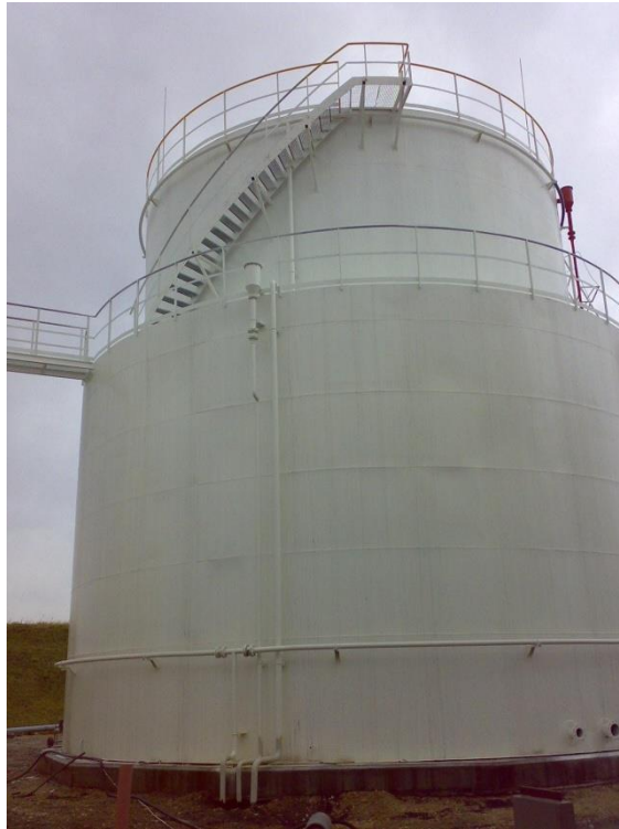
fig. 2 Steel tank with double shell and double bottom
